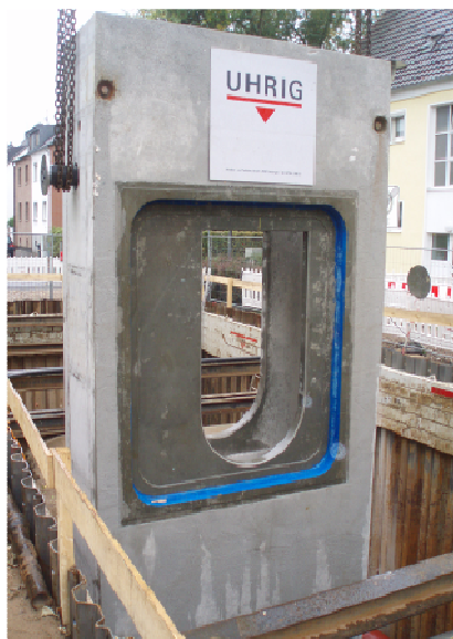
Figure no. 1 – The installation of a mobile dam
