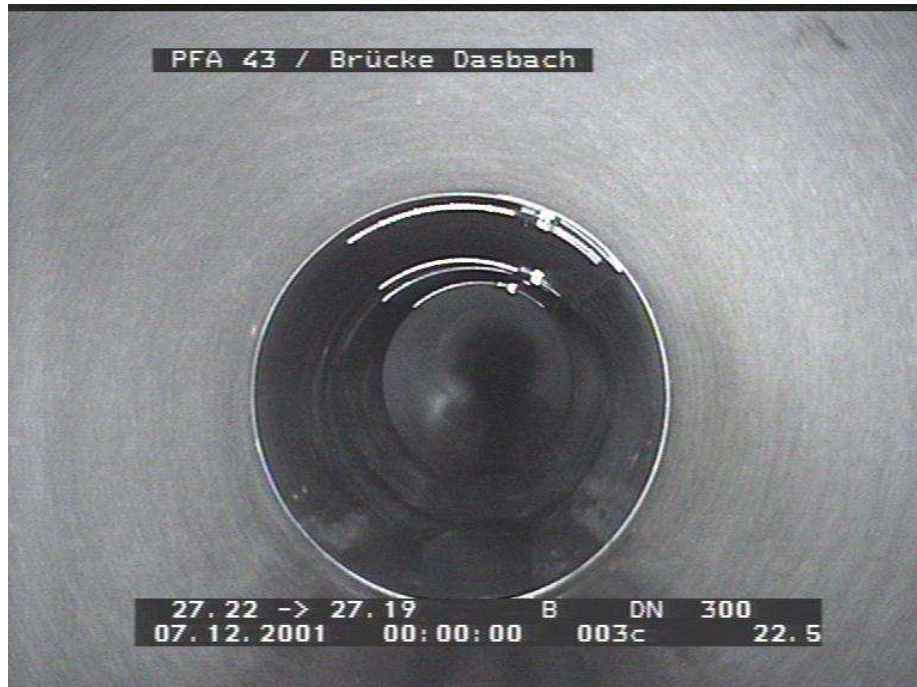
Figure no. 4 – Repaired sewage pipe
